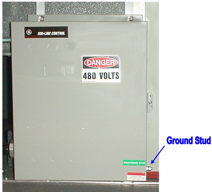
Figure 1: Ground Connection
